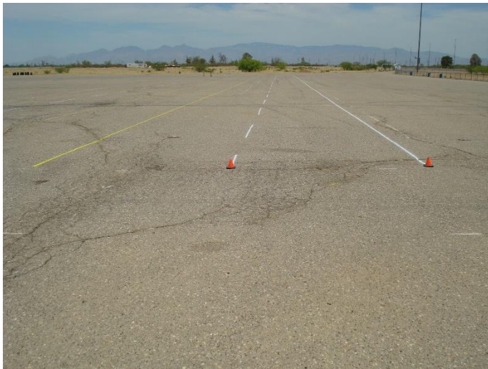
Photo 3. Layout of the two-lane travel way and gate.
