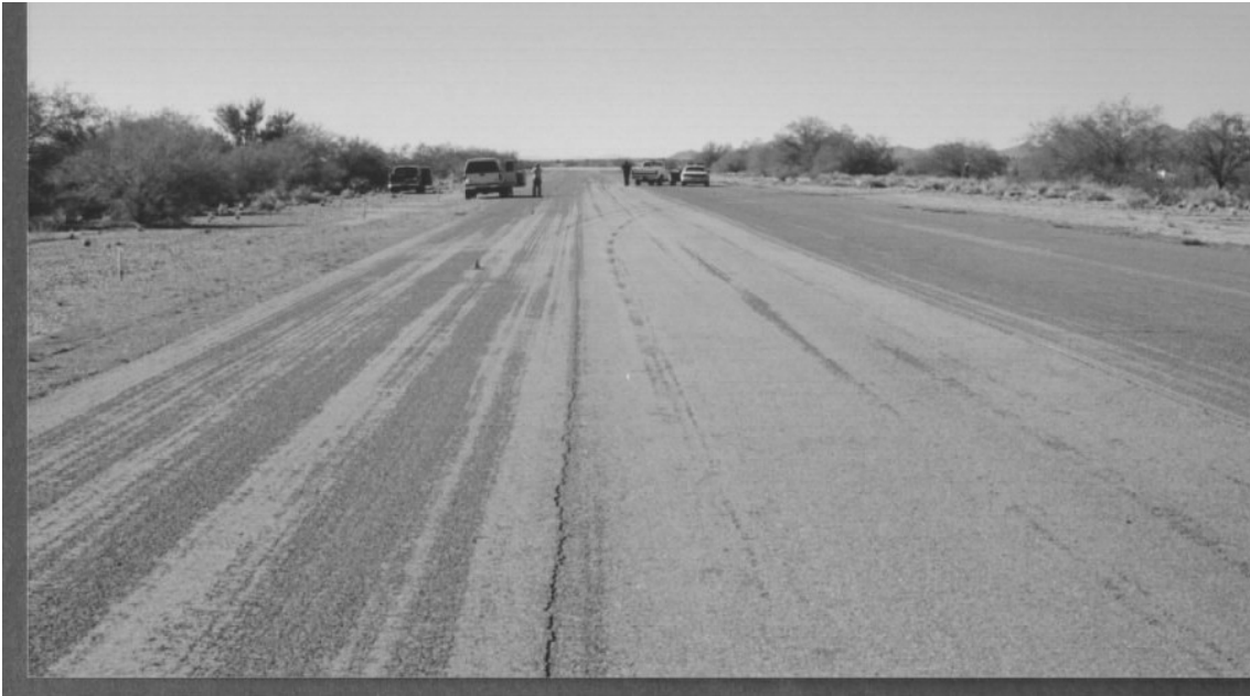
Photograph 1. Start of hopping right rear tire marks
