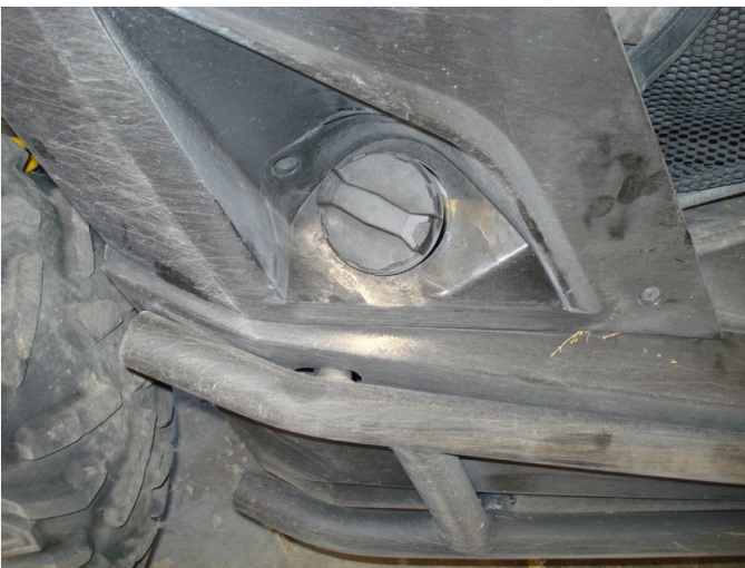
Figure 9. Side structures in close proximity and substantially outboard of the fuel cap.
